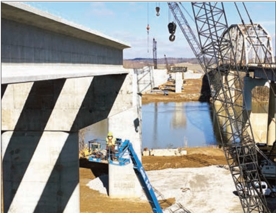
Motorists in the Smithland area of U.S. 60 can expect continued construction zones at the new bridge site where beams are being positioned on the south approach spans. The new bridge will have a 40-foot-wide, two-lane deck with 12-foot-wide driving lanes and 6-foot-wide shoulders, allowing motor vehicles to share the bridge with most farm equipment. The construction schedule calls for moving traffic to the new bridge in spring 2023.
